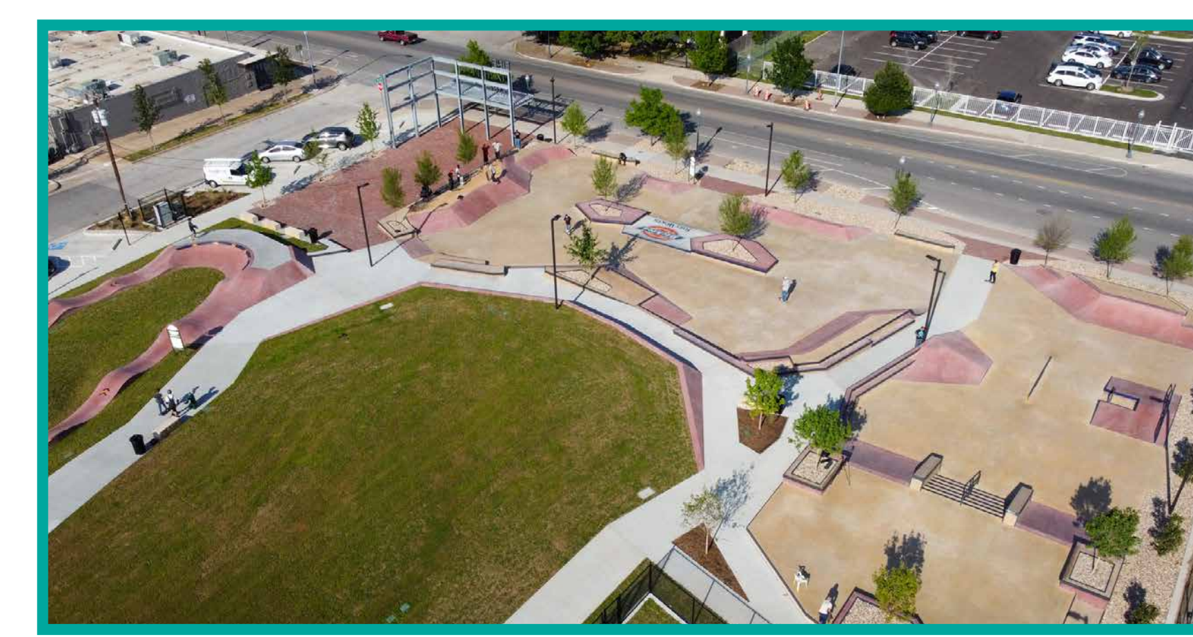
Fire Station Skate Plaza Fort Worth, TX
